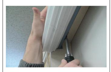
2. Place shade on a flat surface. Remove the dust cover using a flat head screwdriver. Starting with the top corner, run the screwdriver across the top. Put pressure on the back to remove.
