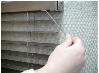
**9.** Adjust the cord stop beads or safety tassel so they are approximately 3" from the bottom of the headrail.
